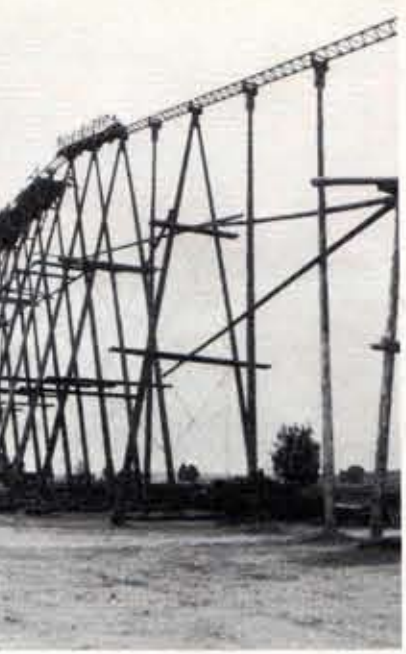
Simple wooden trusses supported track at Schwarzkopf's works in Bavaria, where the teardrop-shaped loop (above) was perfected in 1975. An outgrowth was the Shuttle-Loop (below), in which counterweight or catapult gets train up to speed for forward/backward runs.
