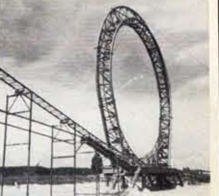
Simple wooden trusses supported track at Schwarzkopf's works in Bavaria, where the teardrop-shaped loop (above) was perfected in 1975. An outgrowth was the Shuttle-Loop (below), in which counterweight or catapult gets train up to speed for forward/backward runs.
