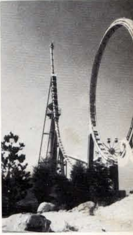
Simple wooden trusses supported track at Schwarzkopf's works in Bavaria, where the teardrop-shaped loop (above) was perfected in 1975. An outgrowth was the Shuttle-Loop (below), in which counterweight or catapult gets train up to speed for forward/backward runs.
