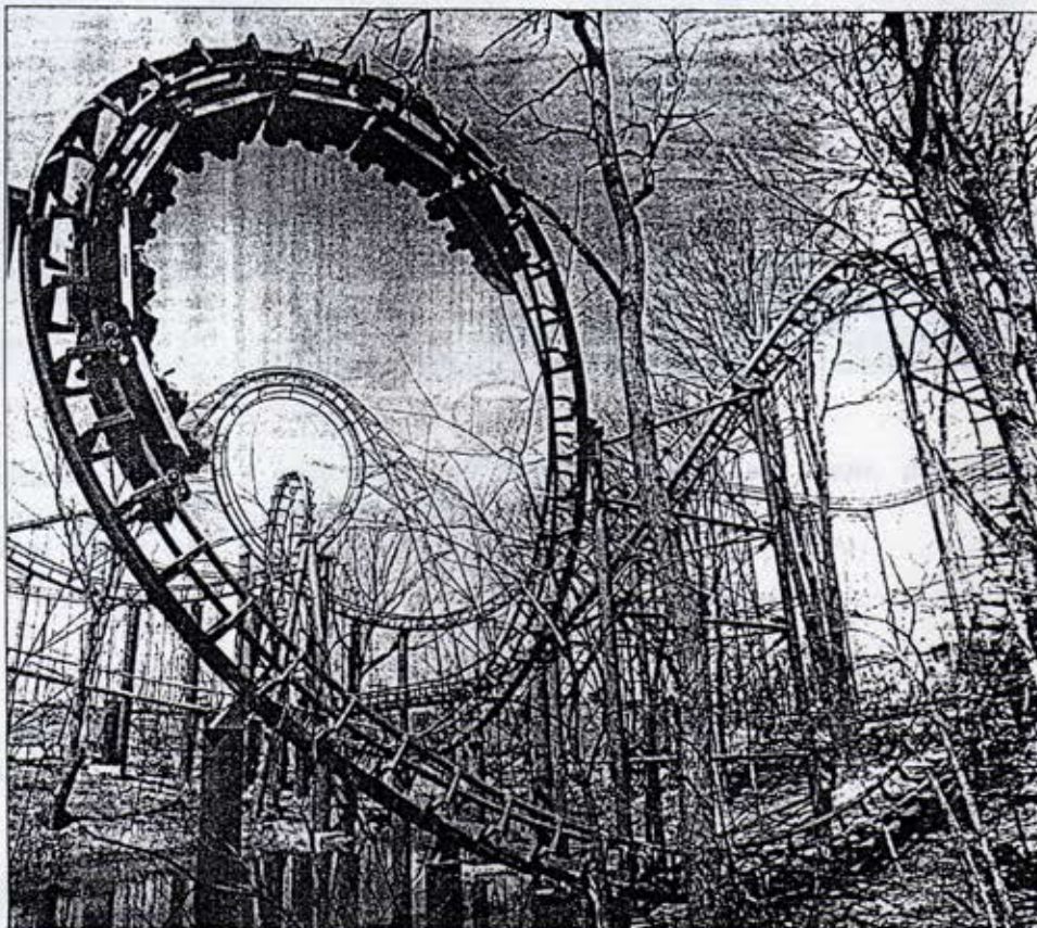
A major attraction at Worlds of Fun is the Orient Express roller coaster. The ride reaches a speed of 65 mph and completes the 3,470 feet of track in about 2 1/2 minutes.
