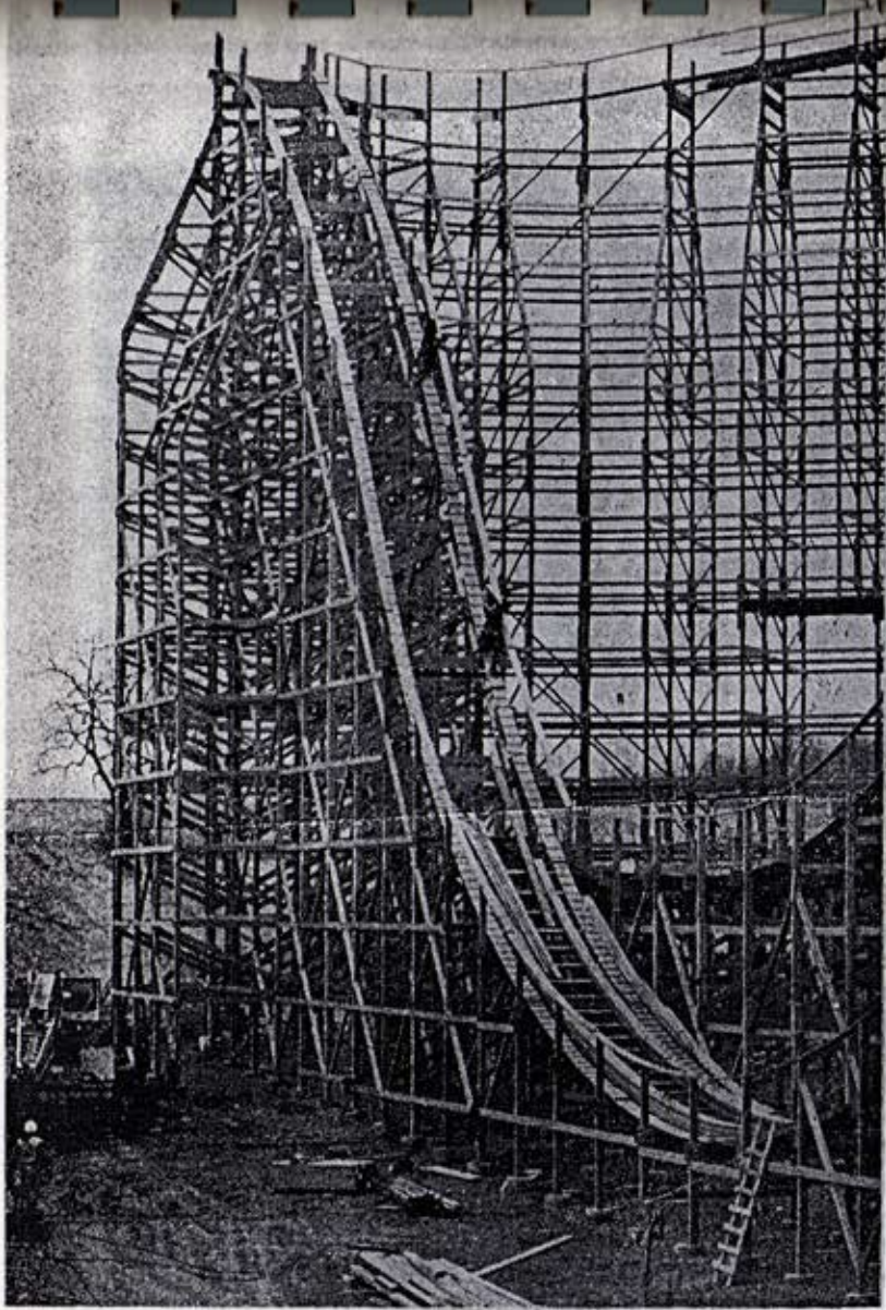
The highest bent is placed 100 feet above the ground on the giant wooden roller coaster structure currently under construction at Worlds of Fun. The $3 million
